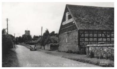
The construction was of oak and brick set on of plinths Totternhoe stone and originally it was thatched. It was tiled in the early 1900's.
